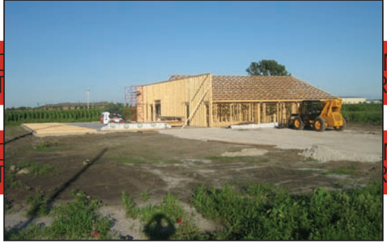
The trusses are in place over the office area.
